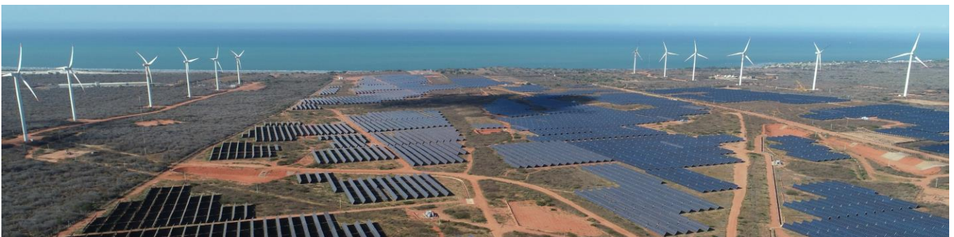
Figure 1. Adjacent power plants located at Areia Branca – RN, Brazil: Floresta 1, 2 and 3 photovoltaic power plant – Engie Solar. Mar e Terra (left) and Areia Branca (right) wind power plants – AES Brasil.
